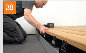
Installation of the last board
