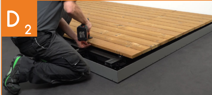
Installation of the boards over an area
