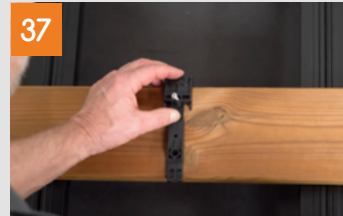
Installation of the last board
