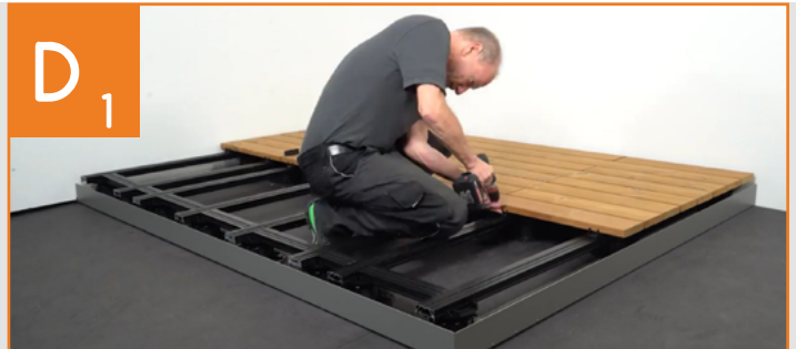
Installation of the boards over an area
