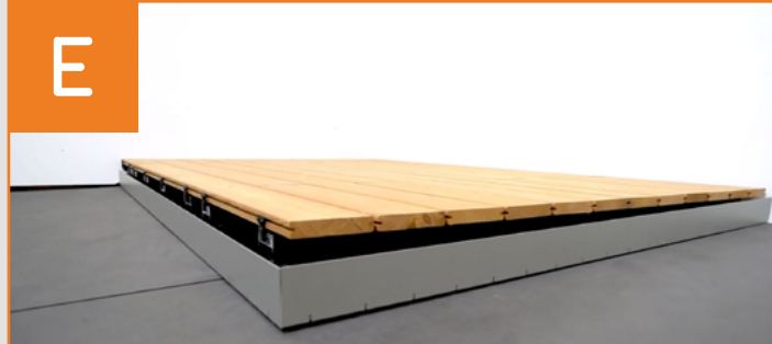
Installation of the last board
