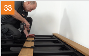
Installation of the boards over an area
