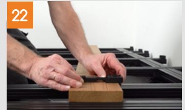
Installation of the first board
