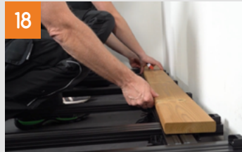
Installation of the first board
