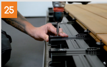
Installation of the last board
