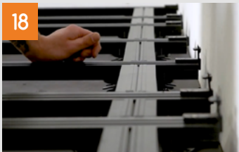
Installation of the first board
