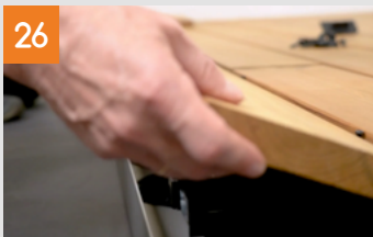
Installation of the last board
