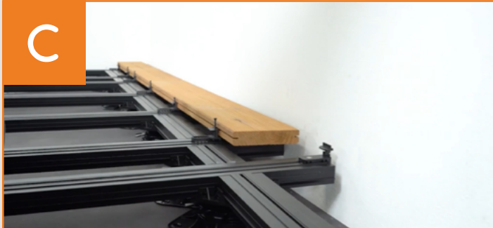
Installation of the first board
