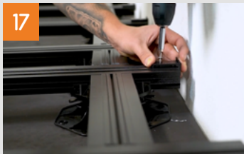
Installation of the first board
